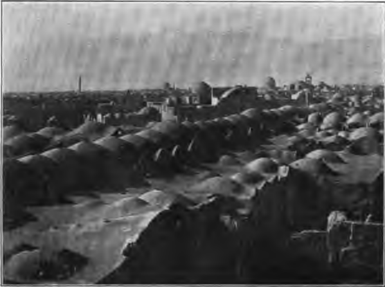
DOMED ROOFS OF KASHAN
